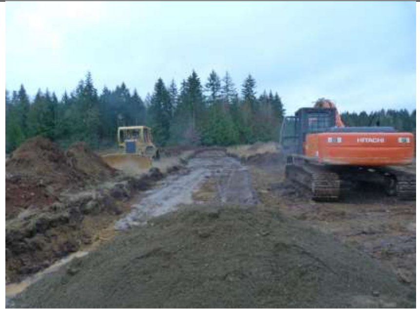
Scraping off topsoil
