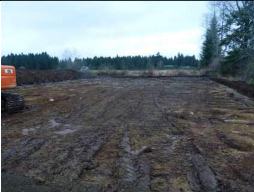
Scraping off topsoil
